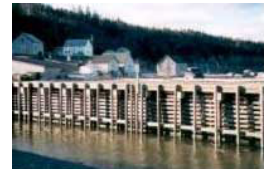
Hall's Harbor - World's first fully composite reinforcement Warf
