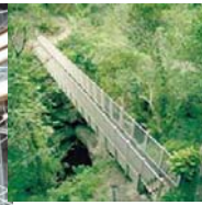
Full bridge Structures (Parson's Bridge, Whales)
