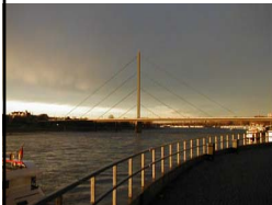
Ulenbergstrasse Suspension Bridge with FRP tension cables (Düsseldorf, Germany)
