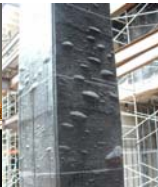
FRP wrap on a column (UF Law School)
